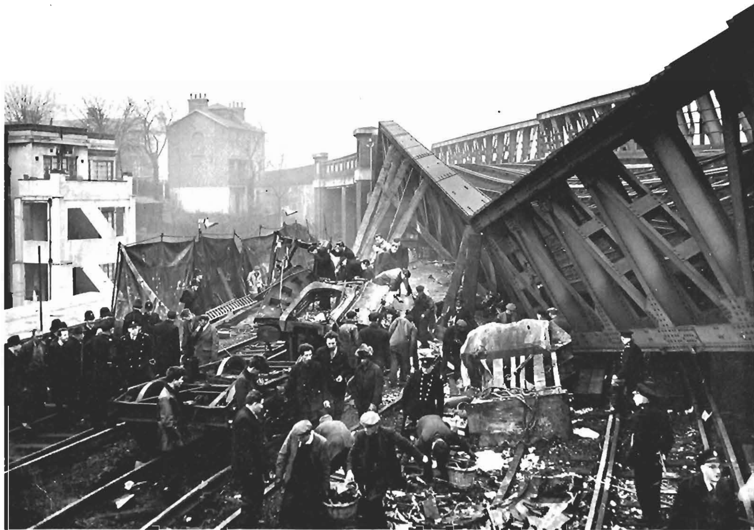
BRIDGE No. 111. AFTER THE ACCIDENT.
